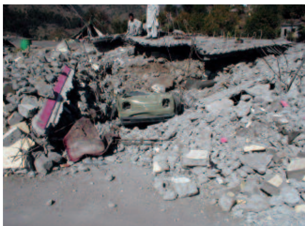
The devastated city of Balakot after the October 8, 2005, earthquake in Pakistan. Approximately 50 journalists based in Balakot, Muzaffarabad, Karachi and Islamabad were identified as killed, missing, injured or directly affected by the earthquake.
